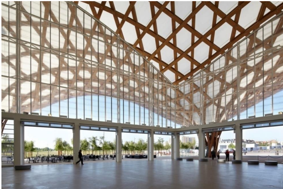
Figure 38: The interior of the Pompidou center in Metz, France, showing the laminated timber structure and the hexagonal pattern of the connections.
